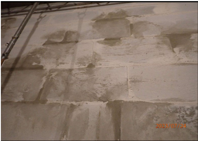
Photograph 23 - P7240497 - 3rd floor roof access storage.
