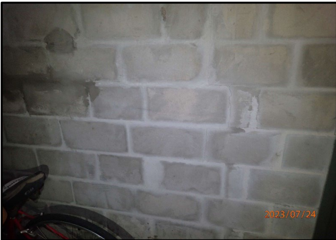
Photograph 11 - P7240424 - EMR wall.
