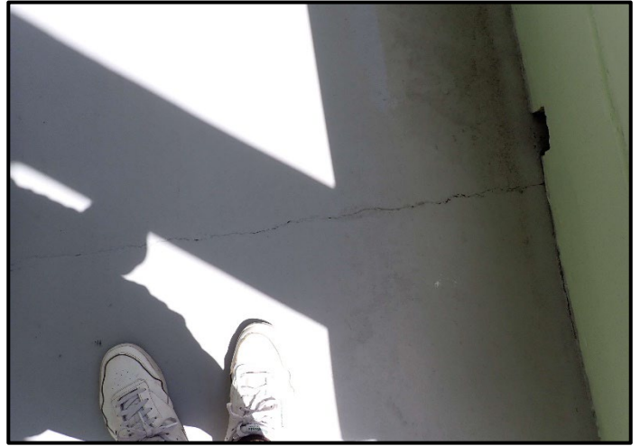
Photograph 06 - P7180595 - 2nd SE wing.
