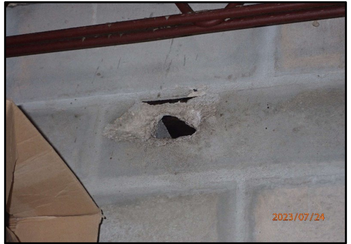
Photograph 16 - P7240453 - 1st storage room.
