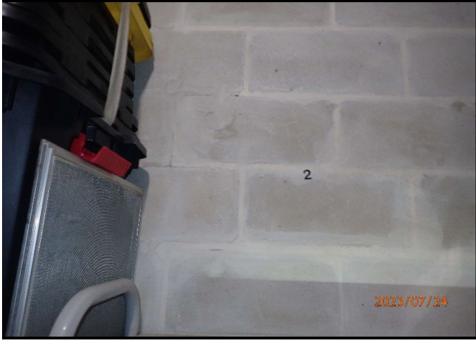
Photograph 17 - P7240454 - 1st storage room.
