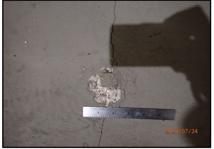
Photograph 14 - P7240442 - electrical room floor.
