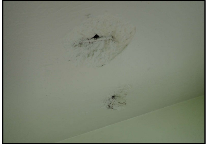
Photograph 10 - P7190016 - stair 1st landing SE wing.
