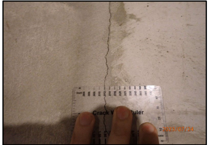
Photograph 22 - P7240478 - 2nd flr large storage room.
