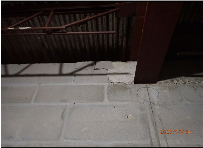
Photograph 19 - P7240459 - 1st storage room
