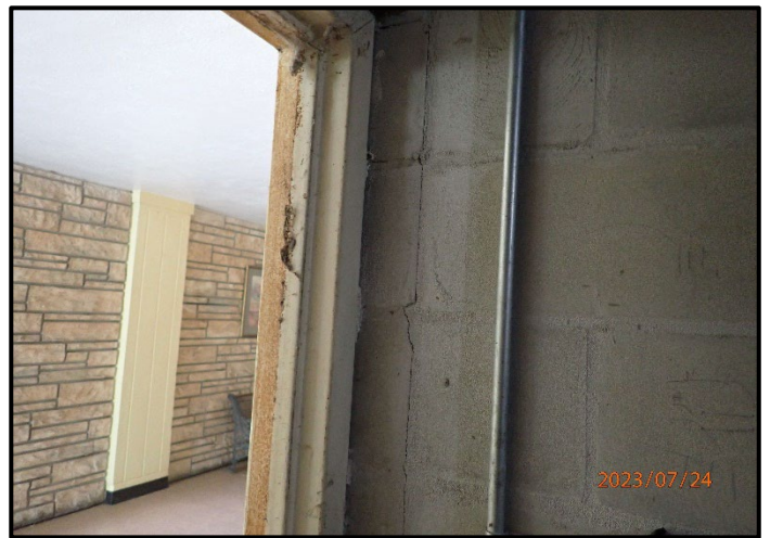
Photograph 20 - P7240461 - 1st storage room
