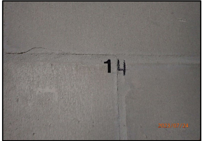
Photograph 18 - P7240457 - 1st storage room.
