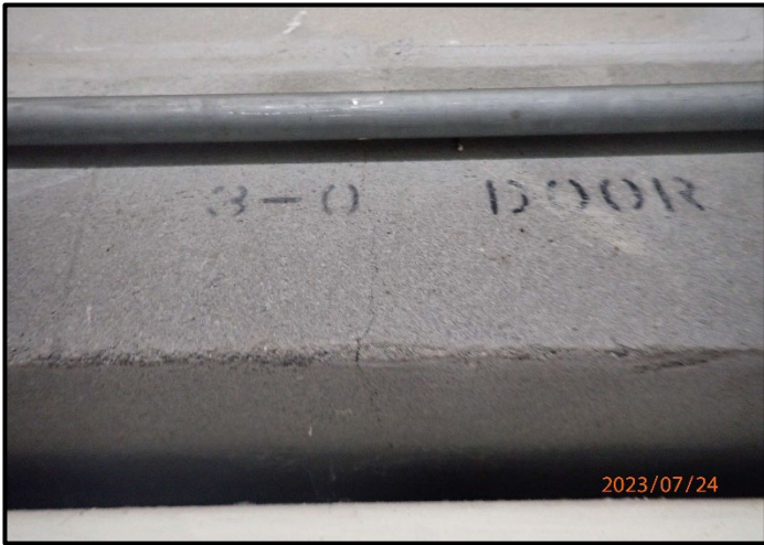
Photograph 15 - P7240445 - electric room lintel.
