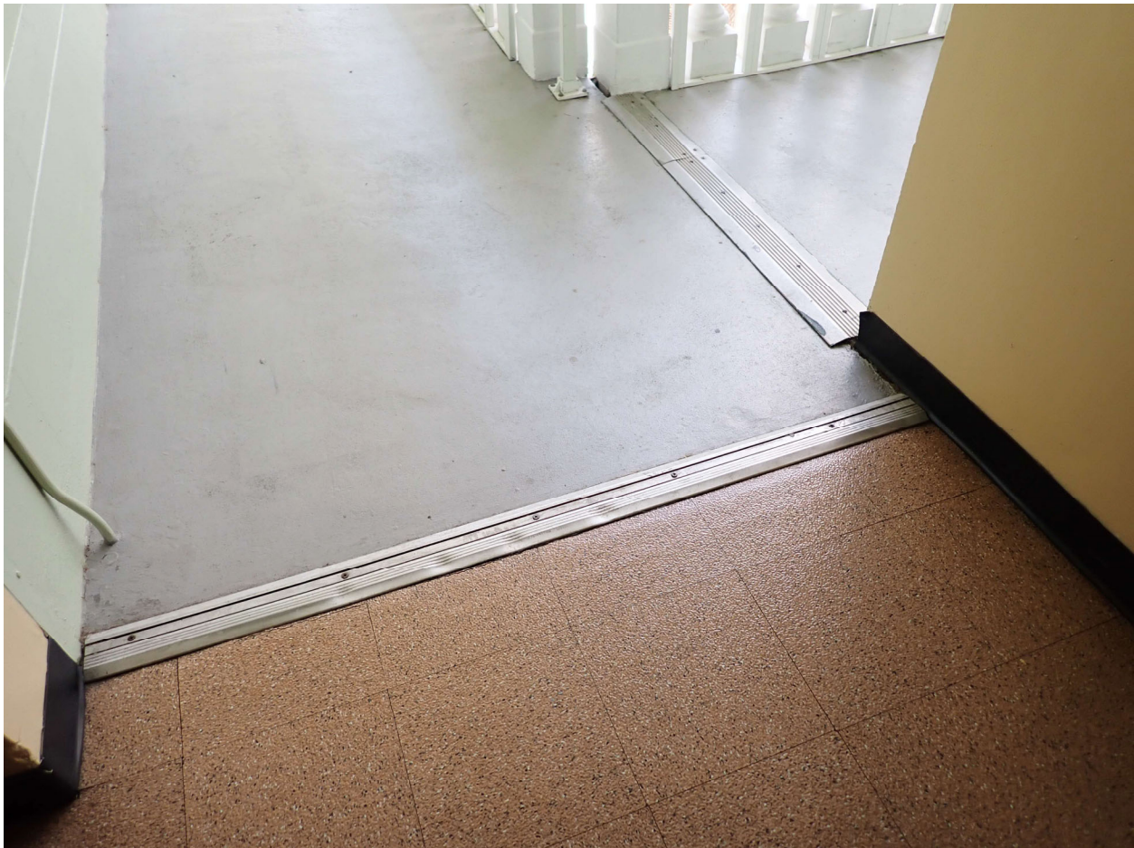
Figure 5. Representative expansion joint at wing/core intersection.
