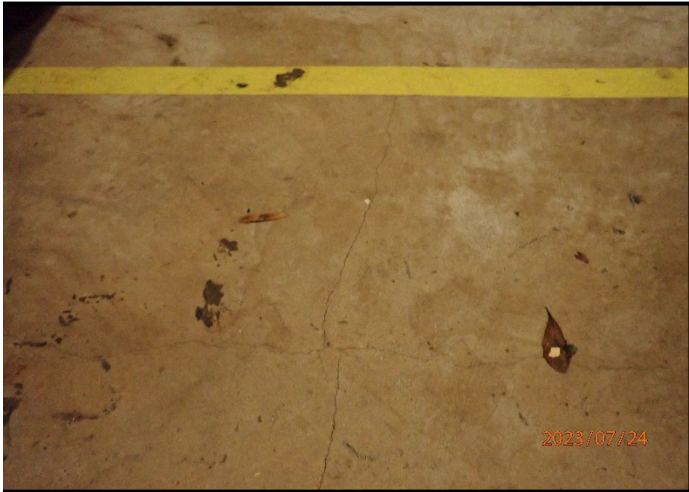
Photograph 21 - P7240471 - 2nd flr small storage room.
