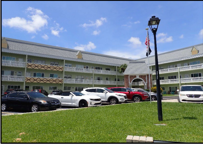
Photograph 01 - P7180457 - front elevation of subject building.
