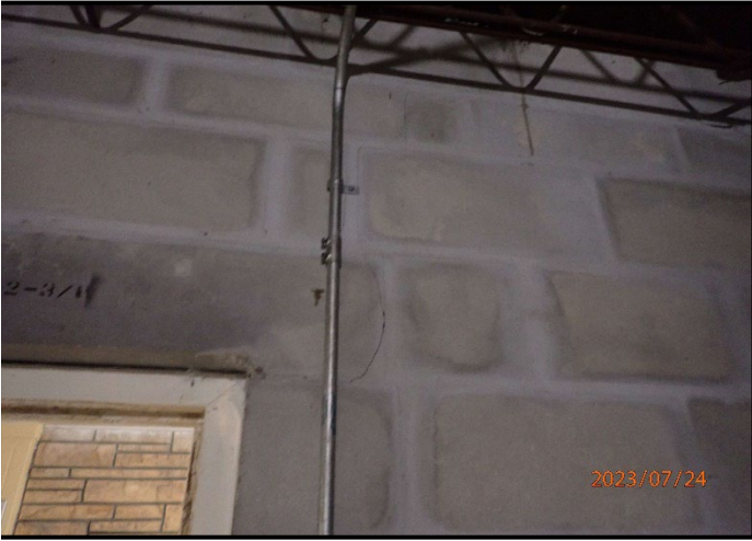
Photograph 13 - P7240429 - EMR door lintel.
