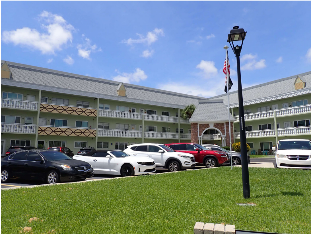
Figure 2. South elevation (front elevation of even units) of subject building.
