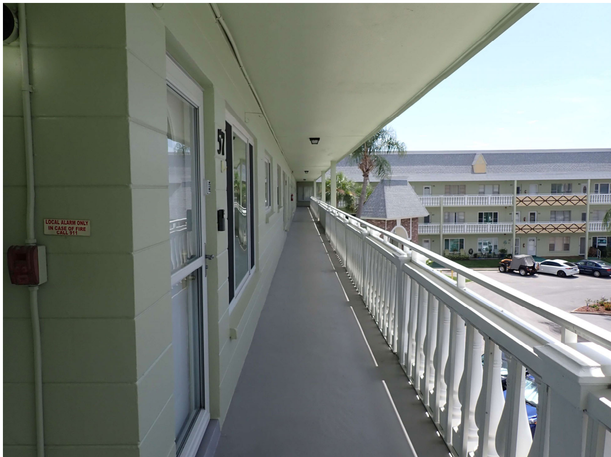
Figure 4. Exterior walkway as constructed.
