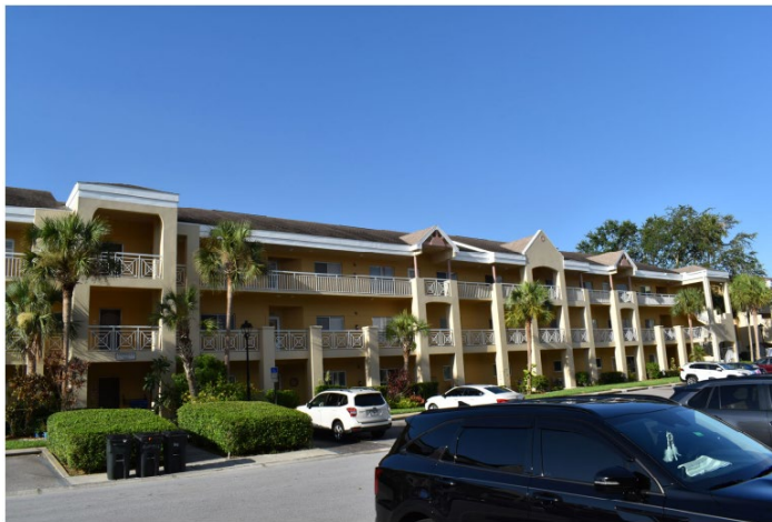
Figure 2. North elevation (front elevation, all numbered units) of subject building.
