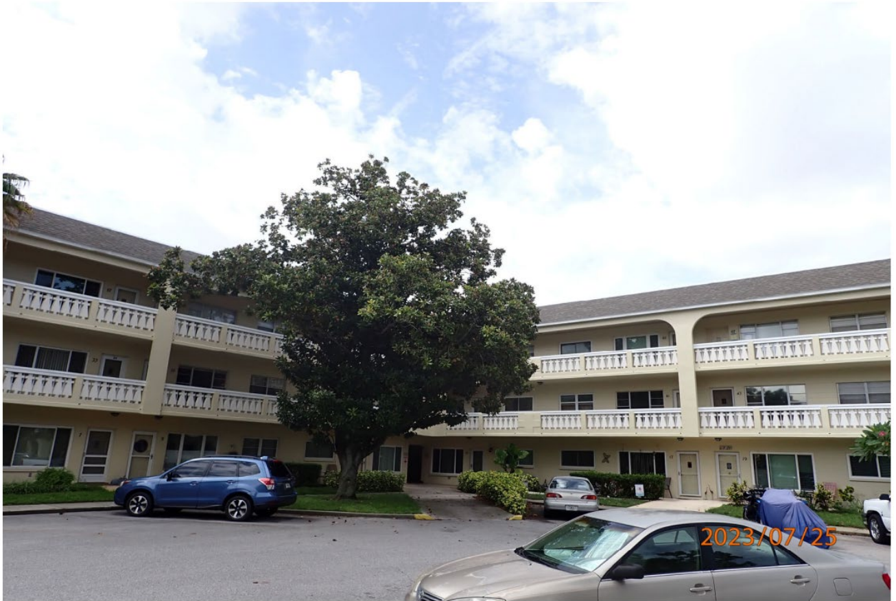
Figure 2. North elevation (front elevation of odd units) of subject building.
