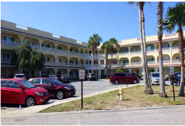
1 Front of Building 85
