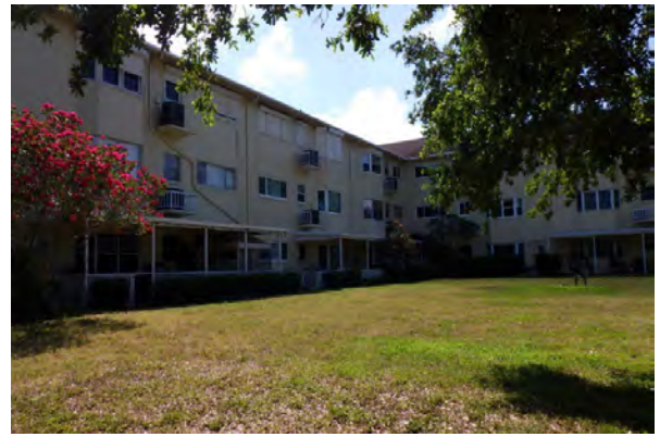
2 Right Side of Building 85
