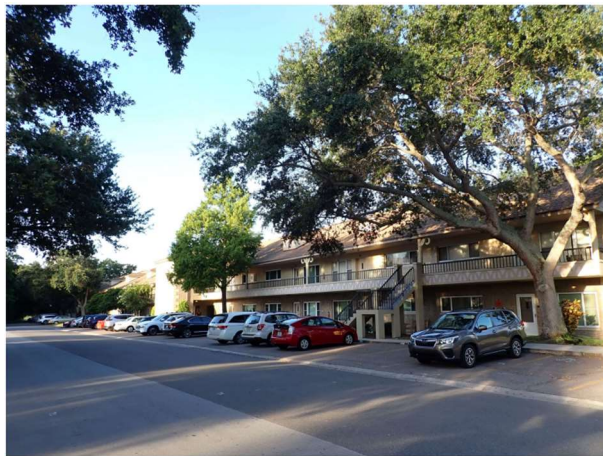
Figure 2. East elevation (front elevation, all even numbered units) of subject building.
