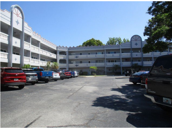
1 Front of Building 73
