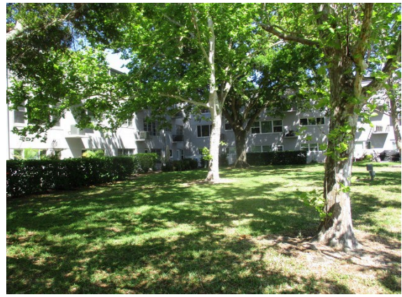
2 Right Side of Building 73
