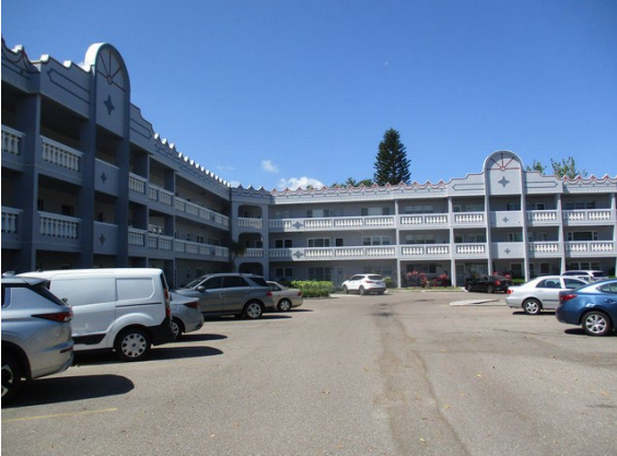
3 Rear of Building 73
