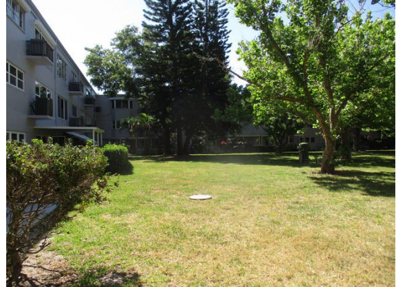
4 Left Side of Building 73
