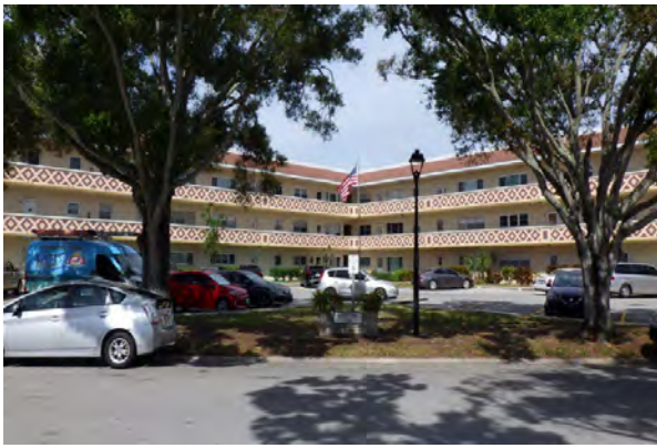
1 Front of Building 61
