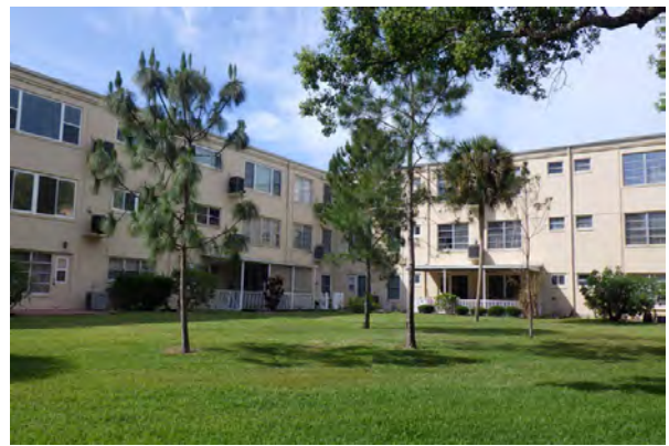
2 Right Side of Building 61
