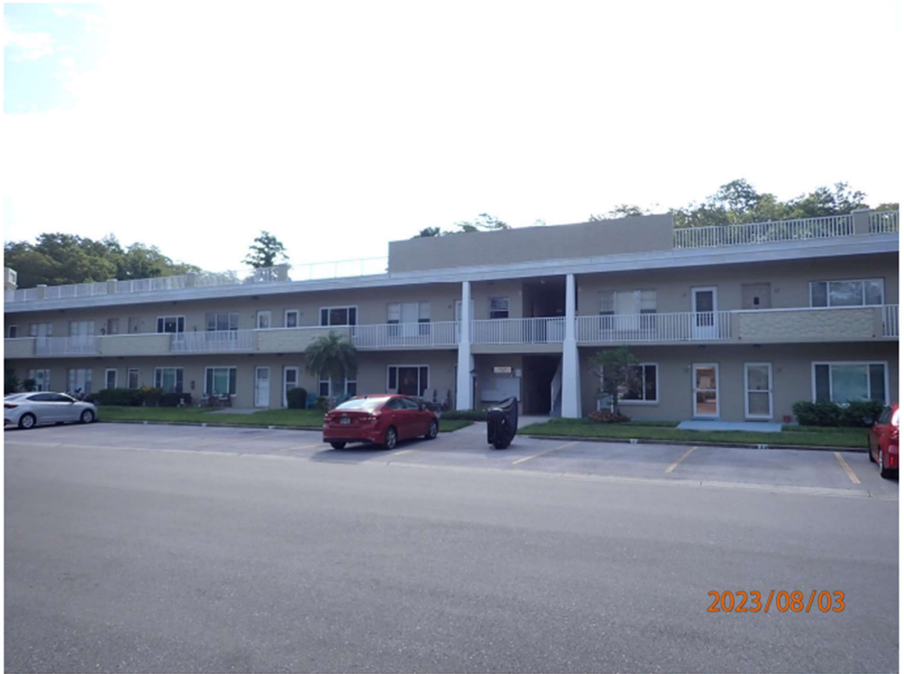
Figure 2. West elevation (front elevation, all numbered units) of subject building.
