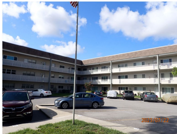
Figure 2. North elevation (front elevation of odd units) of subject building.
