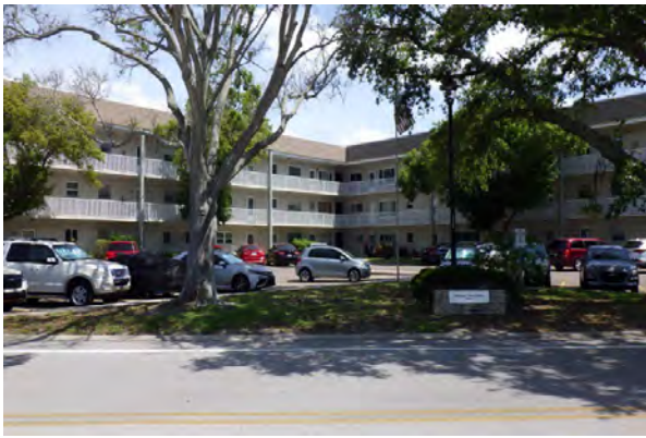
1 Front of Building 54
