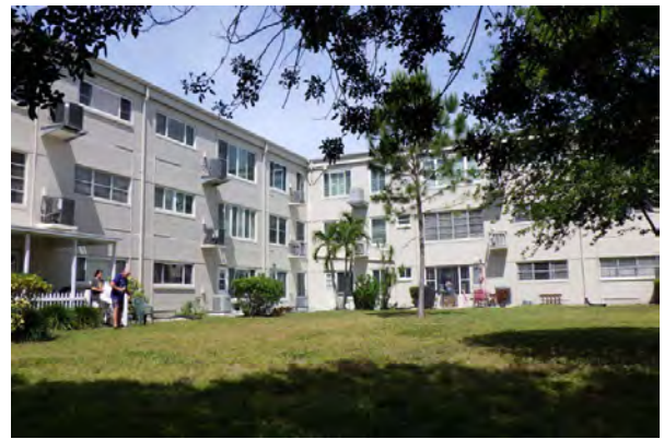
2 Right Side of Building 54
