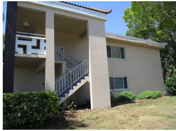
2 Right Side of Building 46
