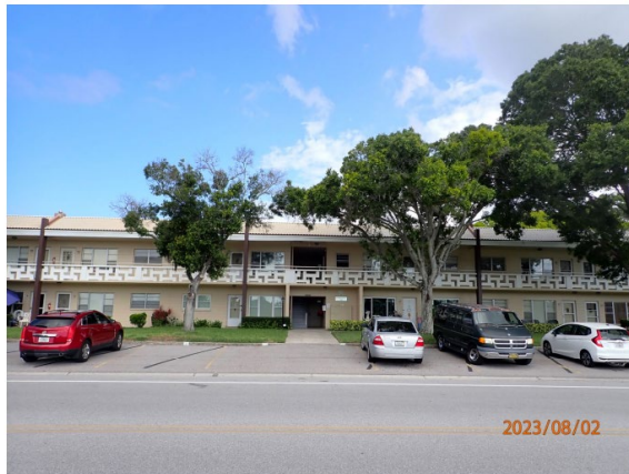
Figure 2. Southeast elevation (front elevation, all even numbered units) of subject building.
