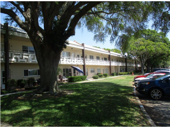
1 Front of Building 46
