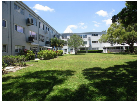
2 Right Side of Building 36
