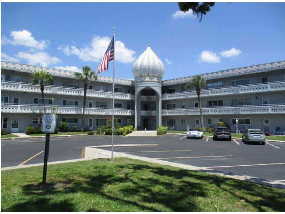
1 Front of Building 36
