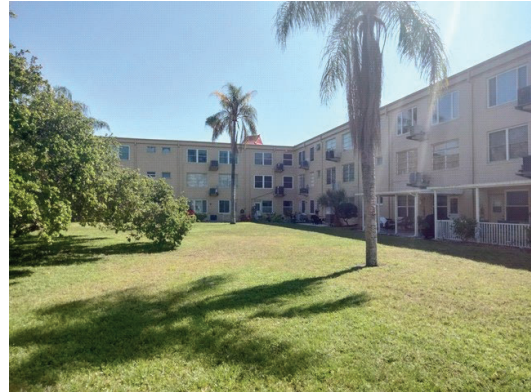
4 Left Side of Building
