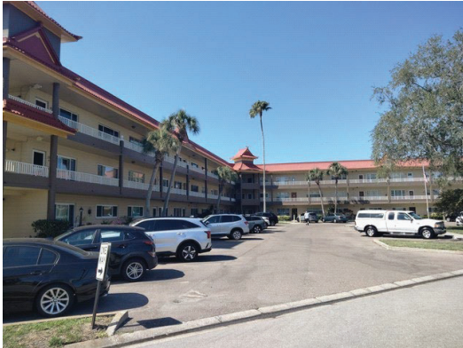
3 Rear of Building
