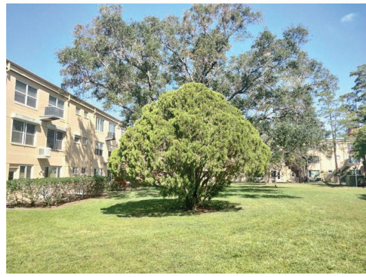
2 Right Side of Building
