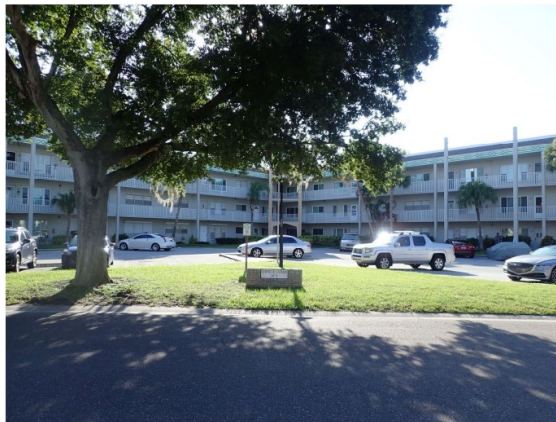
Figure 2. West elevation (front elevation of odd units) of subject building.
