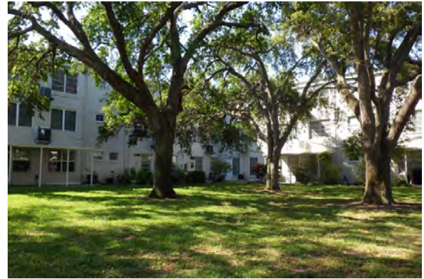
4 Left Side of Building 15
