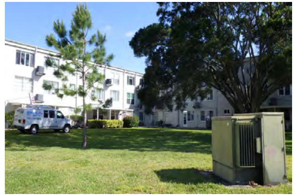
2 Right Side of Building 15
